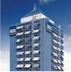
BERU office building at the headquarters in Ludwigsburg
